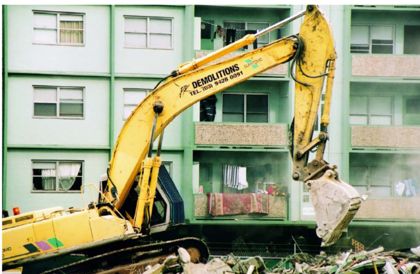
Scenes of the demolition phase, Kensington housing estate.
